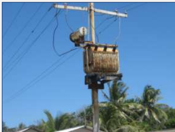
Figure 1. Many of our assets urgently need repair
